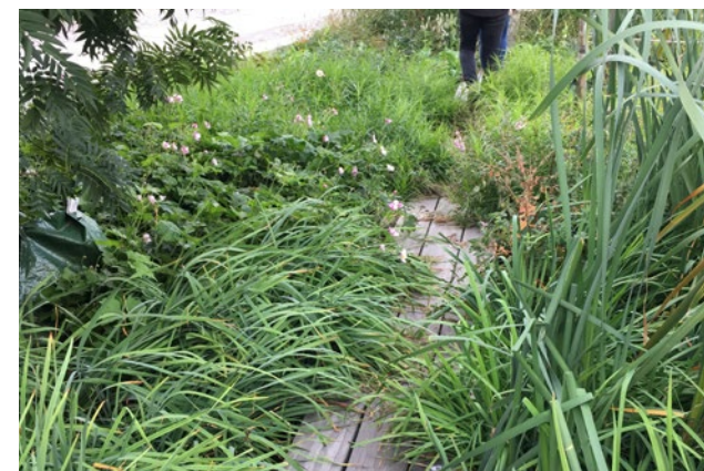
Figure 53: Example of SuD designed as a public amenity and filly integrated into the design of the public realm, Stockholm
