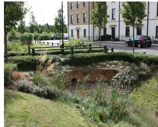
Figure 52: Example of swales check dam integrated with a crossing point, somewhere in UK
