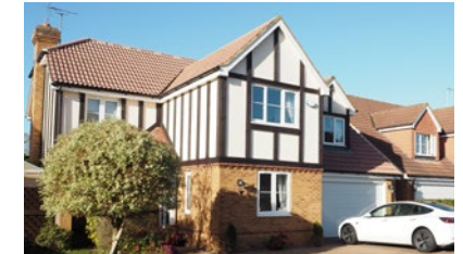
Half timber framing and half render combined with yellow bricks
