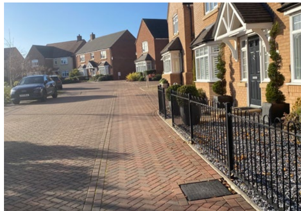
Figure 09: An example of one of the modern residential roads in a development off Station Road
