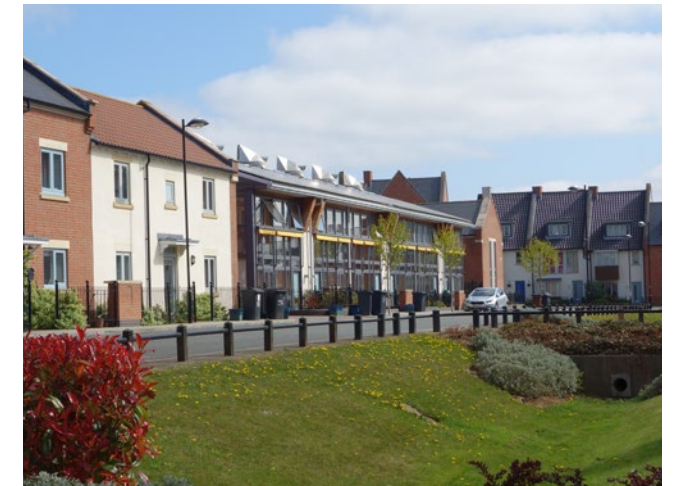
Figure 49: An example of a SuDS corridor - Upton Urban Extension, Northampton
