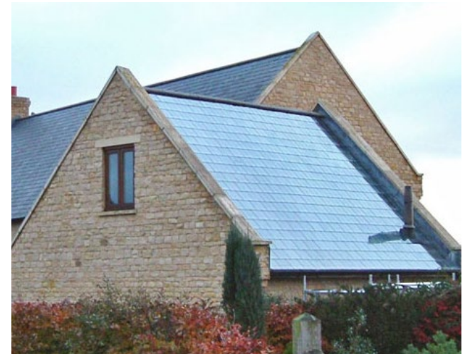
Figure 80: Positive example of implementing solar panels since the design stage.
